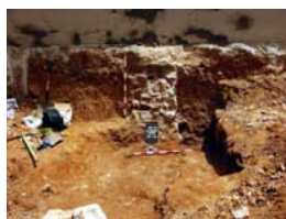
PIC01790 Vista frontal mur u.e. 1144
